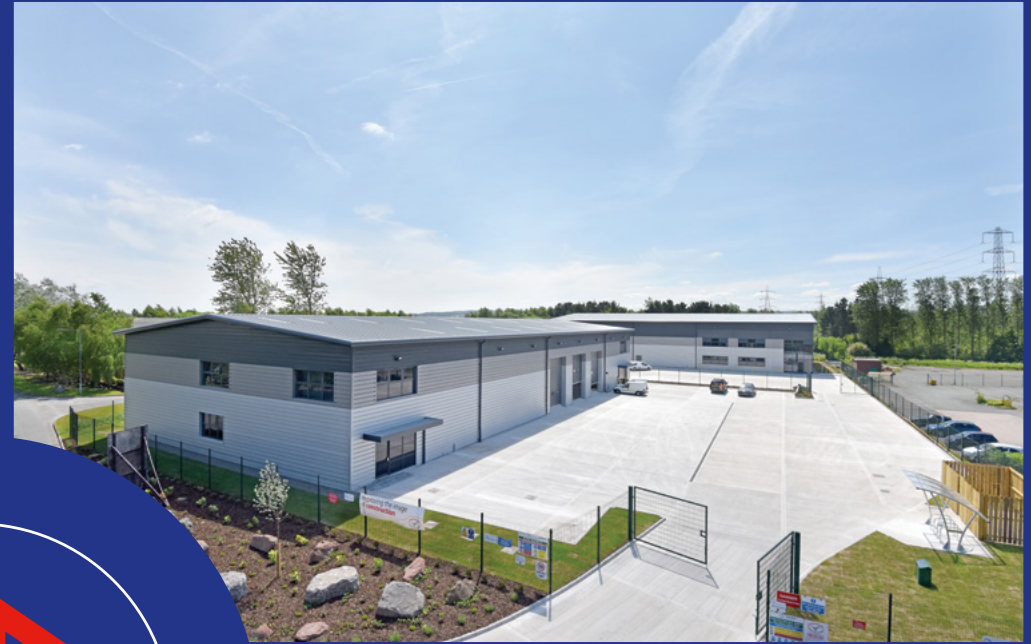
Photography taken Spring 2017 prior to Tenant occupation
