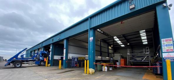
The subjects comprise of a detached industrial unit with yard which is of a steel portal frame construction with a pitched insulated roof incorporating translucent roof panels which was replaced by the tenant in 2021. The walls to the front office section are brickwork with the workshops being rendered blockwork to dado height and clad thereafter.
