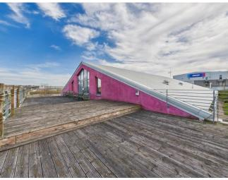
The subjects comprise of a detached unit with the main section being steel portal frame construction with a pitched roof over with the walls being a mixture of rendered blockwork and cladding. The front section is blockwork with a flat roof over with the walls being rendered.
