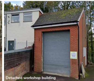
Detached workshop building
